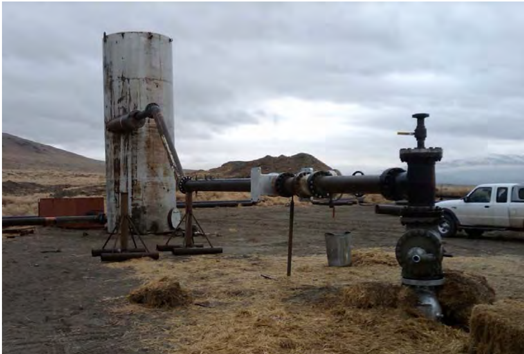
Figure 4-3. Wellhead, flow line, control valve, James tube and atmospheric separator used in geothermal well flow test in Nevada, similar to, but smaller than the separator to be used at Newberry.
